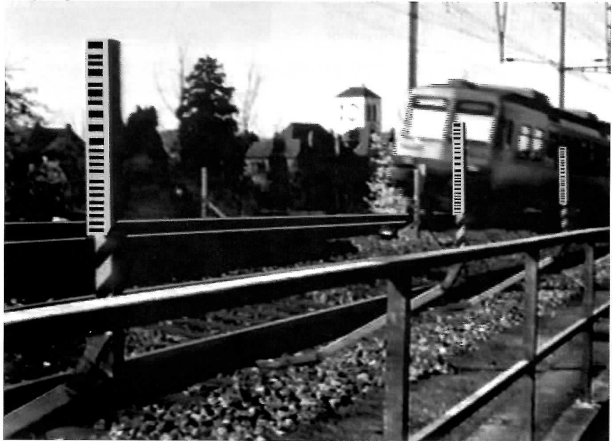
Fig. 2: Bar-code measuring staffs attached -to the train rails along the Lenzburg embankment dam
